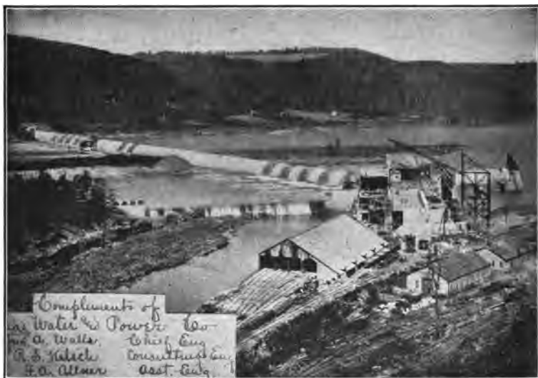
FIG. 102.—Concrete dam built in sections across Susquehanna River, McCall's Ferry, Pa. Power-house and forebay at the right. Tail race sheltered behind island to left. 200,000 horse-power within reach of Baltimore, Philadelphia and Washington. (Penna. Water & Power Co.)
